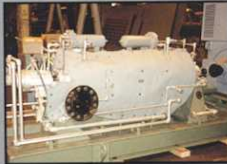
Boiler Feed Water Pump Acoustical Cover
